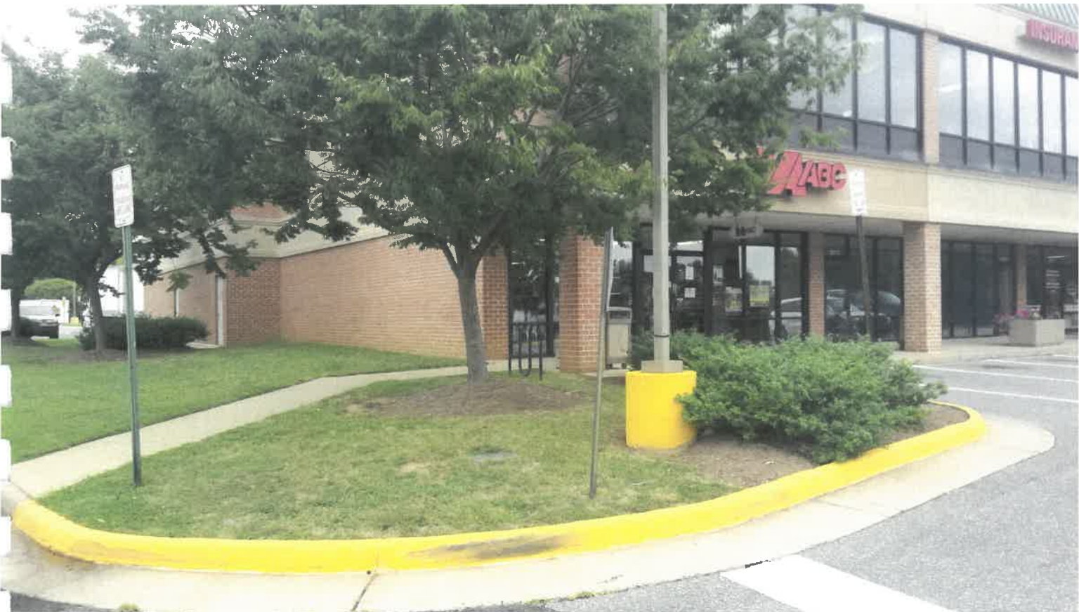
Southeast corner of building
