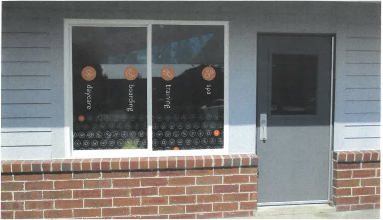
Exterior Hollow Metal Door (20 GA Minimum) w/ Half Lite – Painted Sherwin Williams #SW7075 “Web Gray”
