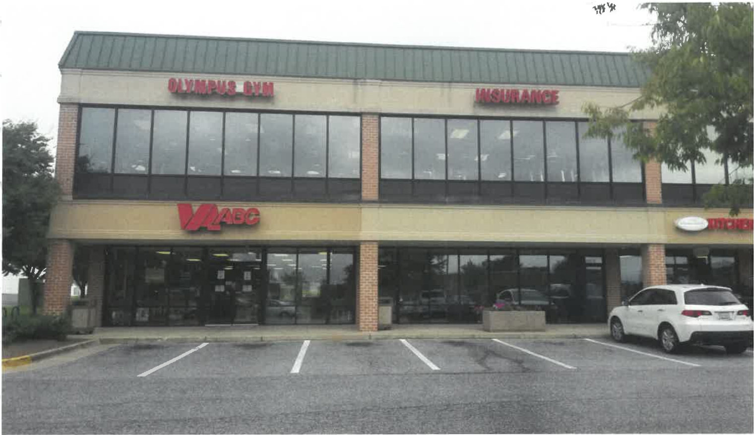
Front of Purcellville Plaza (east side of building)
